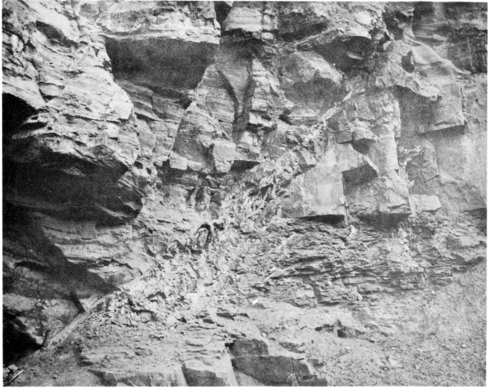
Figure 1 The small fault at the north-east corner of the south-east face of Swancar Quarry. Well jointed Coal Measure sandstones can be seen below the fault; soft red and yellow sandstones above.
